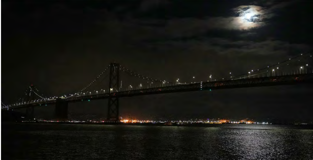
Figure 3. Photo from the New York Times taken in March 2023, showing the Bay Bridge during the period when The Bay Lights had been turned off. The decorative lights on the suspension cables were added in 1986 1 . Although the bridge was lit, as necessary for public safety, the amount of sky-glow was clearly far lower than when The Bay Lights had been in operation.
