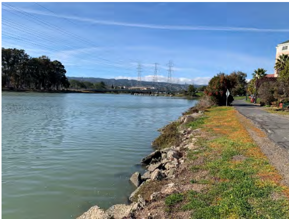
Photo 3. Burlingame Lagoon, south of and adjacent to the site, is channelized with an armored shoreline.
